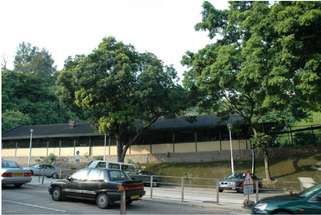
Car park of HACare Home in 2004 (Source: Jao Tsung-I Academy)
