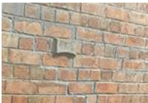
Crack monitors can be found in low zone (Source: Jao Tsung-I Academy)
