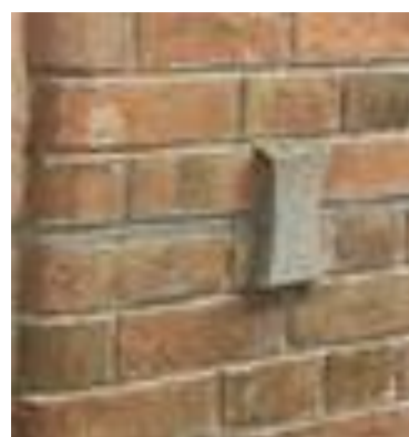
Crack monitors can be found in low zone (Source: Jao Tsung-I Academy)
